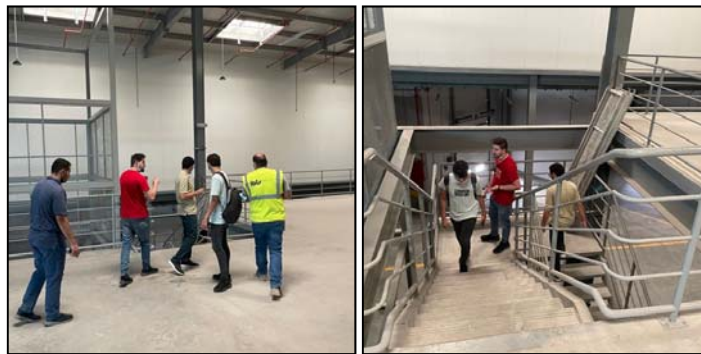
Figure 53 – Construction site visit on October 9, 2021
