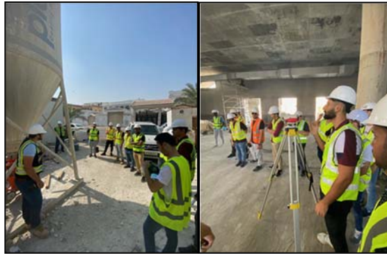
Figure 52 – Construction site visit on November 2021
